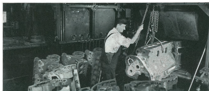
Mack cylinder blocks keep their shape. Shown here, the reason why. Castings enter huge electric furnace for 12 hours of heat treatment. This exclusive process relieves casting strains, prevents distortion.
